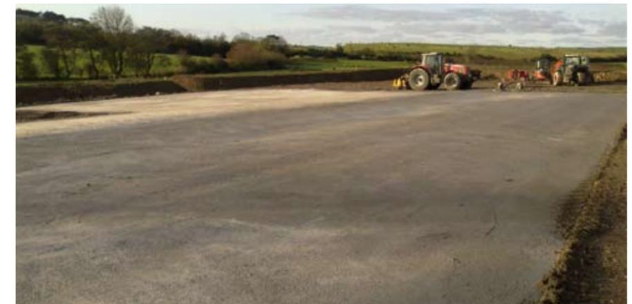
The use of Stehr stabilisation equipment to create the hard standing for enterprises such as biogas plants is a service that has grown over the past year.
