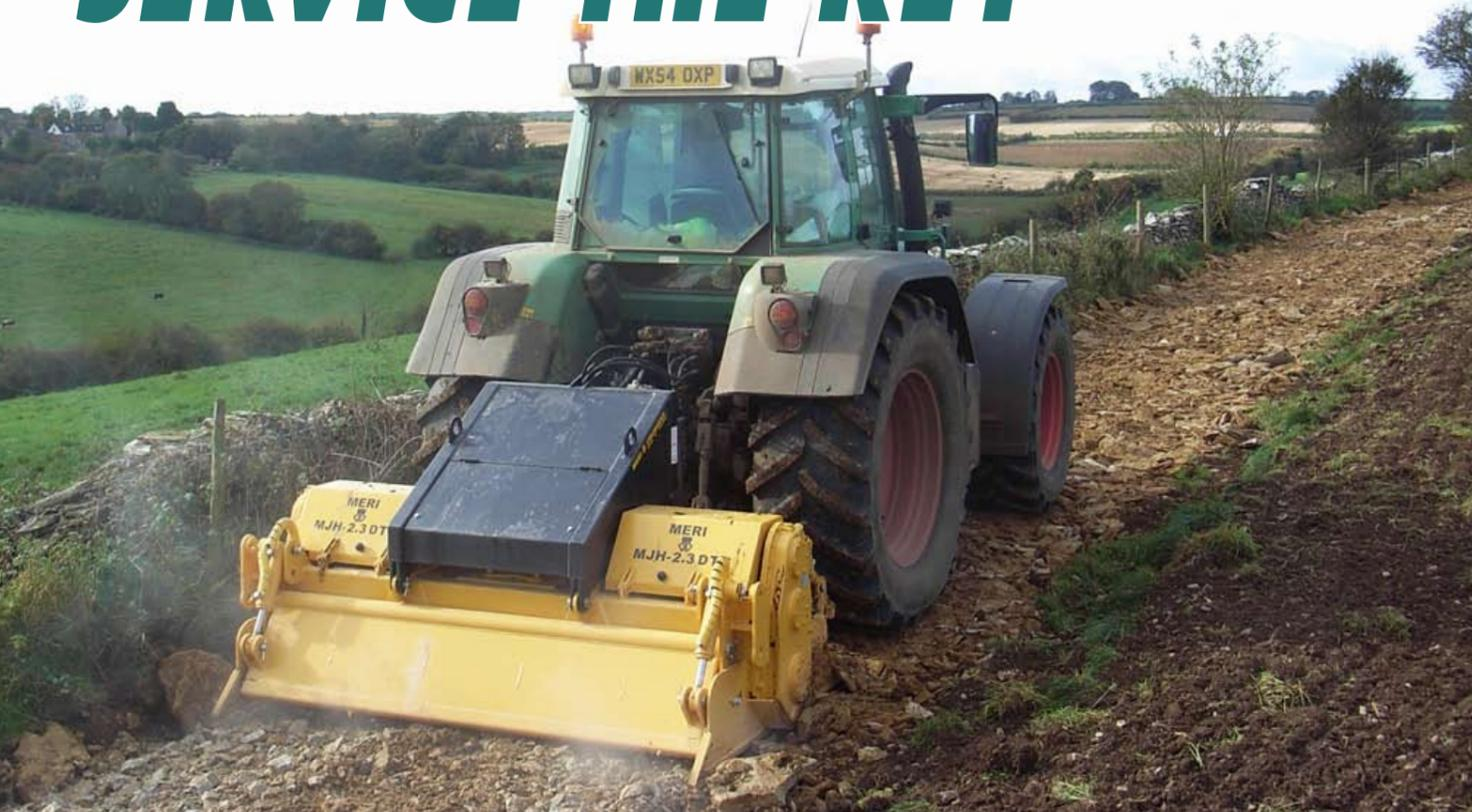
Track restoration with a Meri crusher, the first step of a technique that recycles material in-situ and results in a long-lasting surface.
